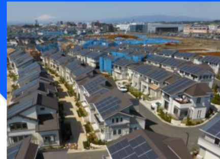
Solar cells, storage batteries and ENE-FARM* installed as standard in each dwelling
