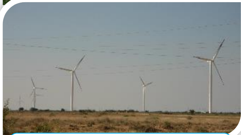
Vayu1 150 MW Wind - Gujarat
